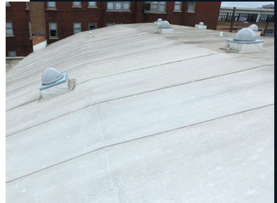
**GREEN GARAGE DETROIT** chose **DURO-LAST** for its roofing membrane because the product satisfied its primary objective—reduced heat absorption in warm months. It reflects up to 88 percent of the sun's energy, so the building interior requires less energy to be cooled. Additionally, pre-made rack flashings accommodated the thermal panels on the building annex roof, which heat the building in winter.
